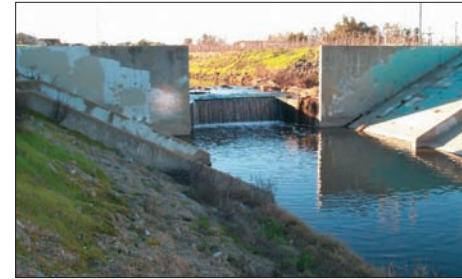
Figure 13 – The Marsh Creek Grade Control Dam Upstream of the Brentwood Wastewater Treatment Plant
