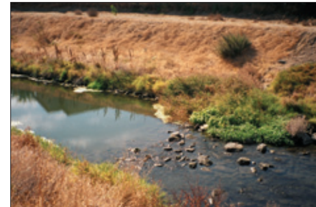
Figure 14 – Grade Control Structures in the Marsh Creek Channel
