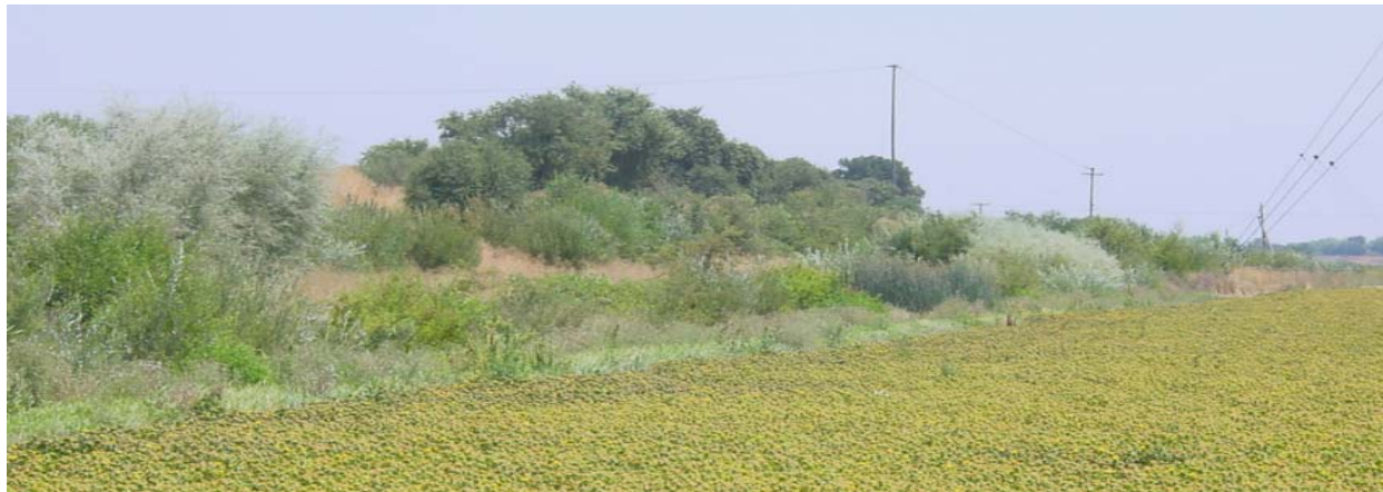
Re-sloped (10-to-1) and re-vegetated levee, with safflower production in the foreground.
