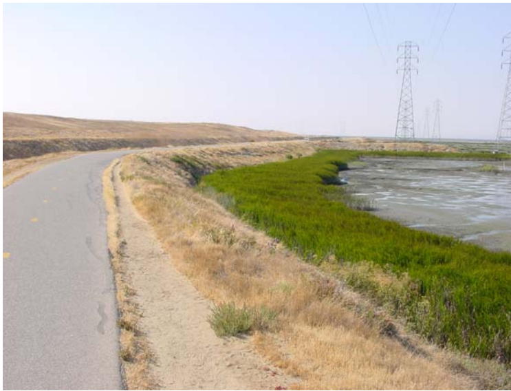
Path along top of levee
