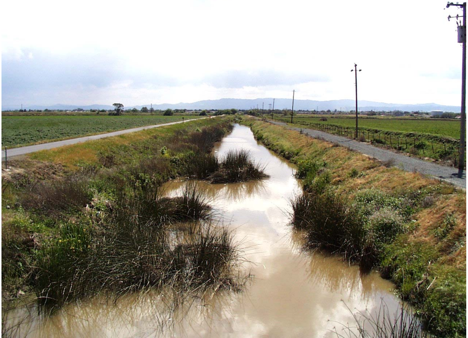
Figure 15. Photo of Marsh Creek channel.
