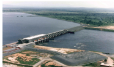
Kpong Dam: 1982, 160 MW
